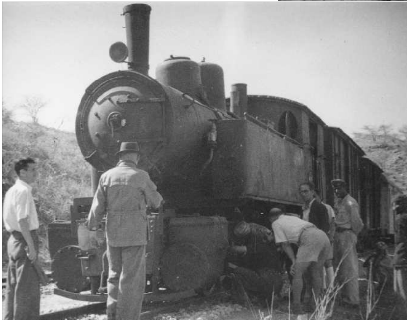
Loco breakdown. John Broughton-Thompson recalled that the motion was dismantled on the low pressure leading cylinder, which meant that one link was distorted and so not functioning properly. Prof Gallo, Chief Engineer, is wearing the hat and Tony Kinsella, the Chief Mechanical Engineer's Assistant, is bending over looking at the distorted link. The Italian man on the left is the driver of the Draisine inspection wagon. Late 1940s.
