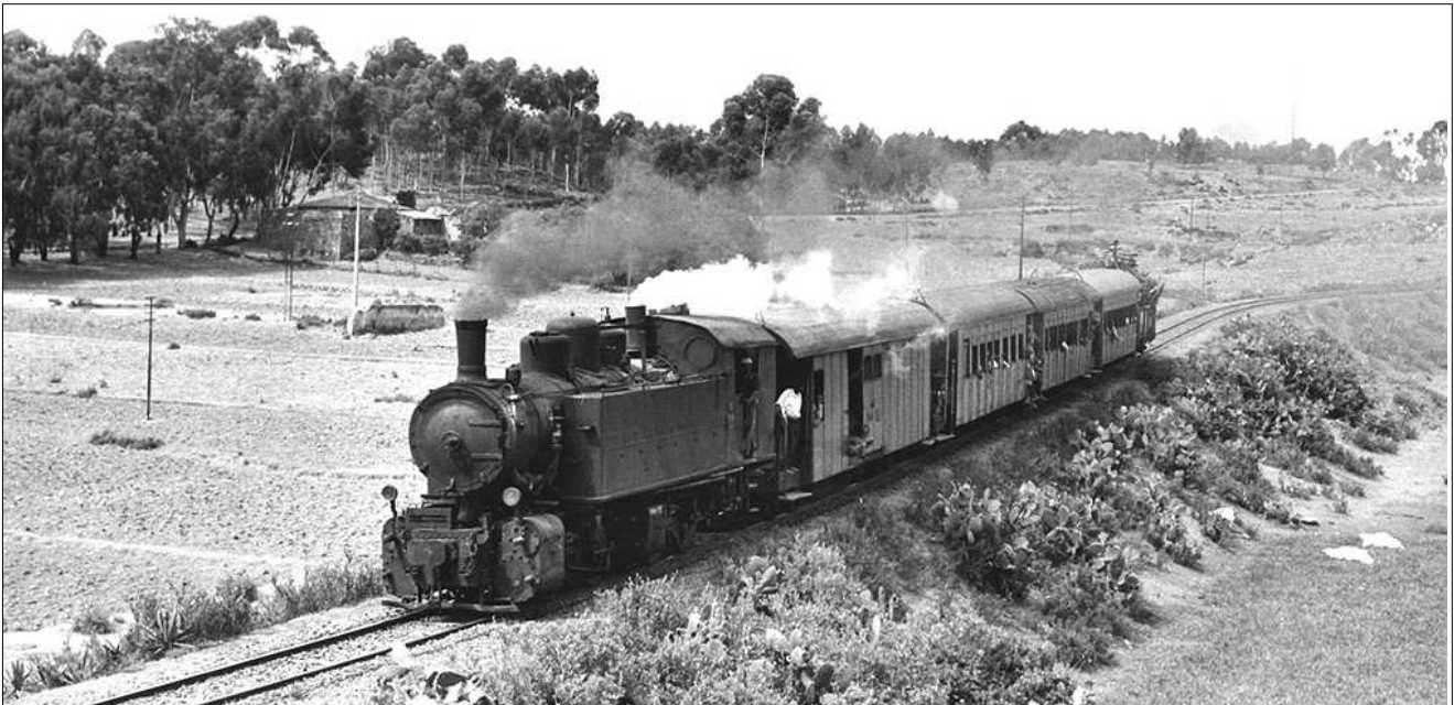
The afternoon passenger train from Massawa approaching Asmara. Notice the passengers hanging out of the windows and a rear wagon piled high with wood. 5 th July 1969
